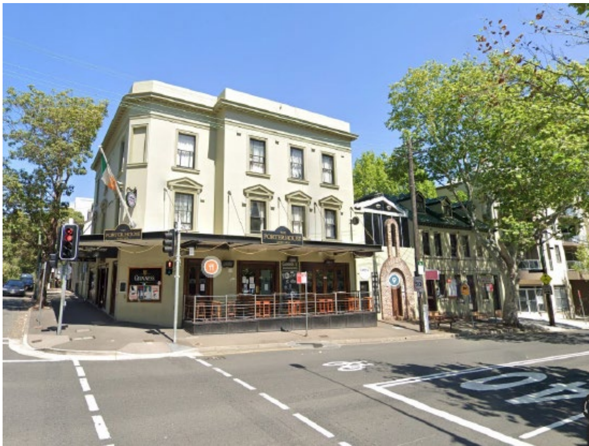
site - Campbell Street
